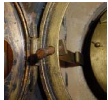
One of the screws holding the movement to the back.
